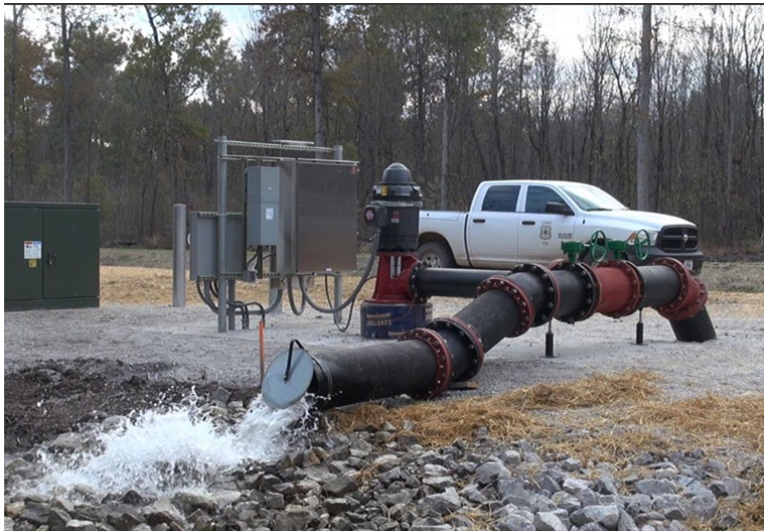
Controlling water levels in a forested wetland (USFS, Shawnee National Forest)
