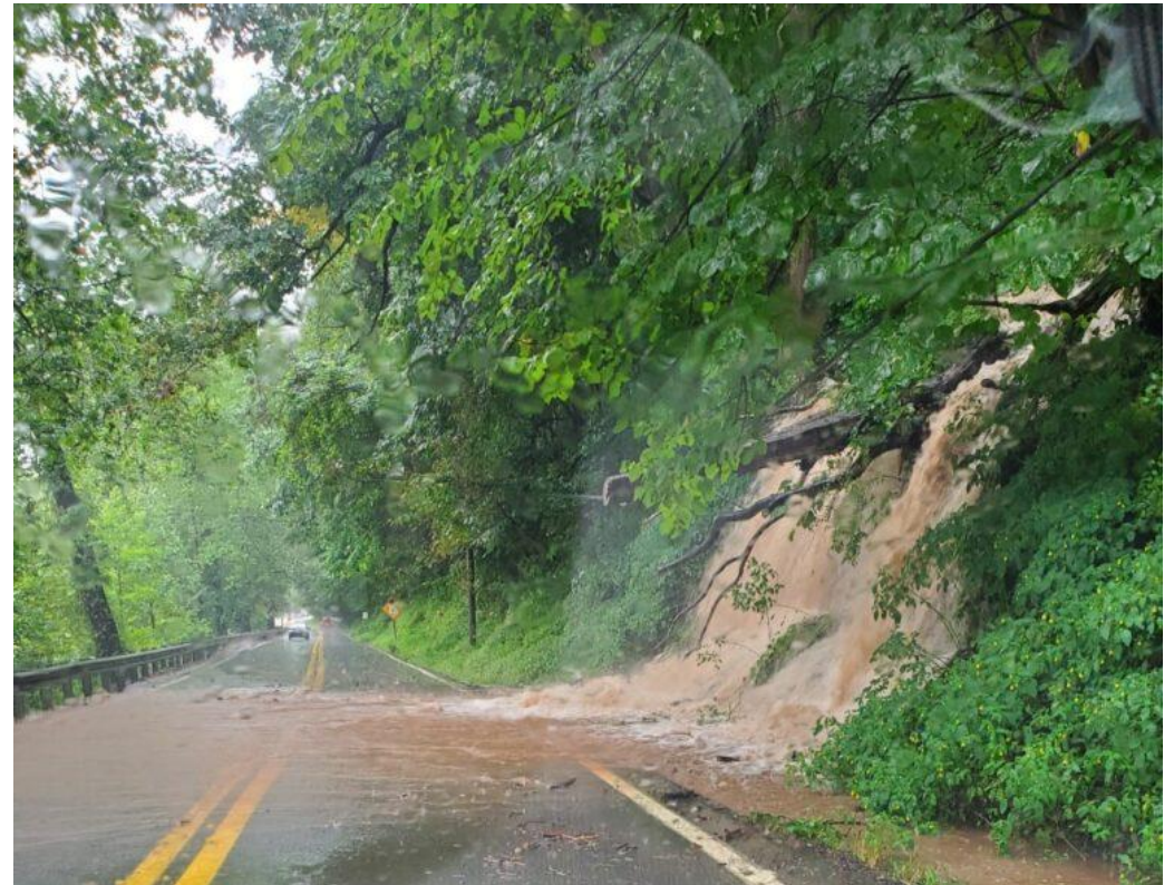
Photo: Route 72 in Preston County
